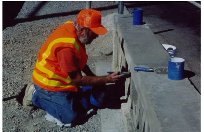
Ellis Nelson applying slip coat
