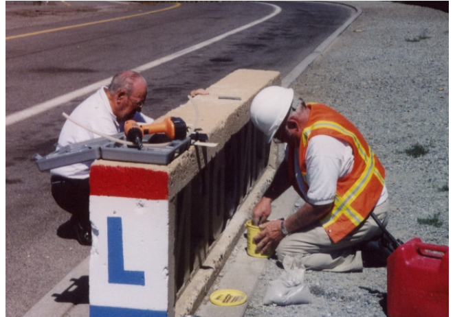
Dustin Ramsey and Norman Root set the new "C" in place
