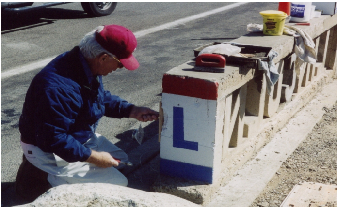
Lloyd Johnson patching concrete
