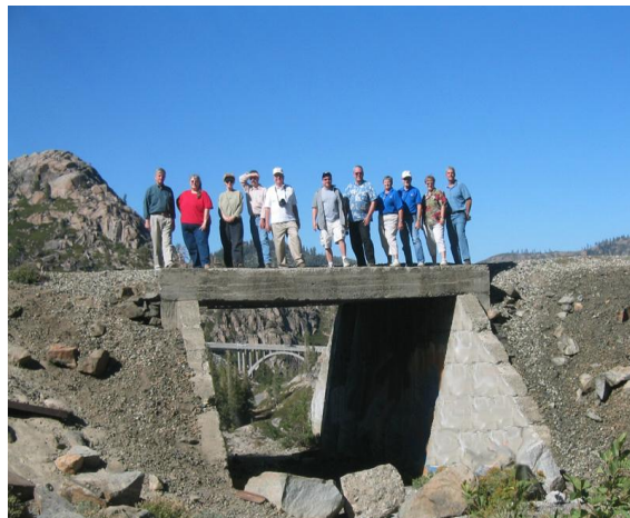
Lincoln Highway undercrossing at Donner Pass
