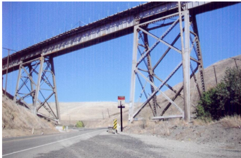
Altamont Pass Road East of Greenville Road E/B- Near Trestle
