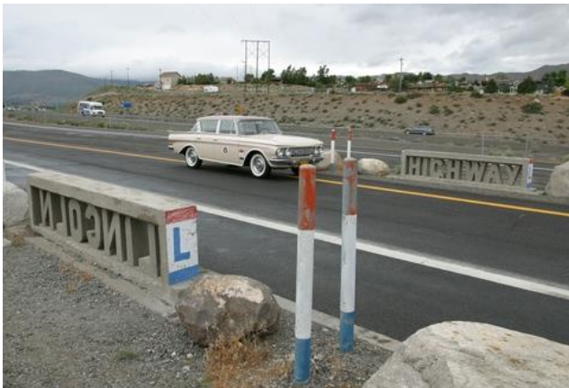
Original bridge railings near Verdi, NV.
