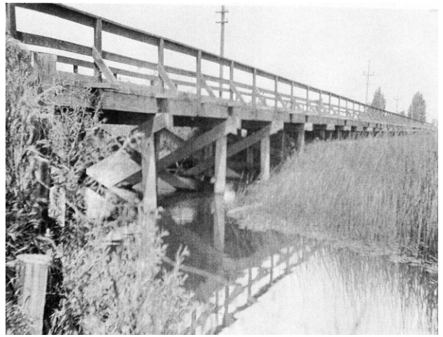
400 foot wooden bridge across Badger Creek 1915
