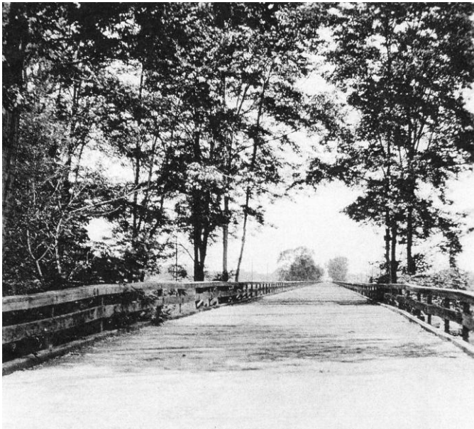
Looking north over 2,300 foot Trestle between the Cosumnes River and Arno.
