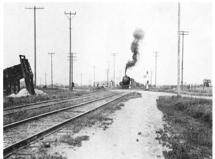
McConnell Station Crossing
