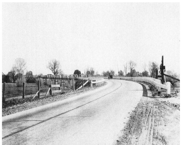
Northern approach to Dry Creek Bridge south of Galt 1925
