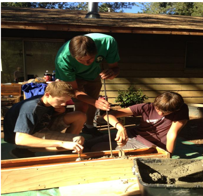
Hand tamping and the use of an oscillating sander helped create the proper finish to the marker
