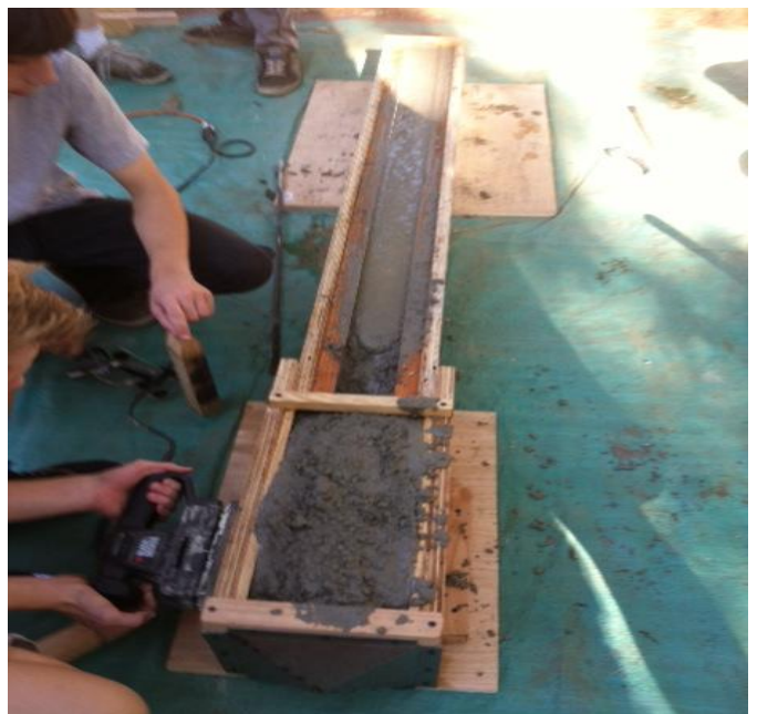
Hand tamping and the use of an oscillating sander helped create the proper finish to the marker
