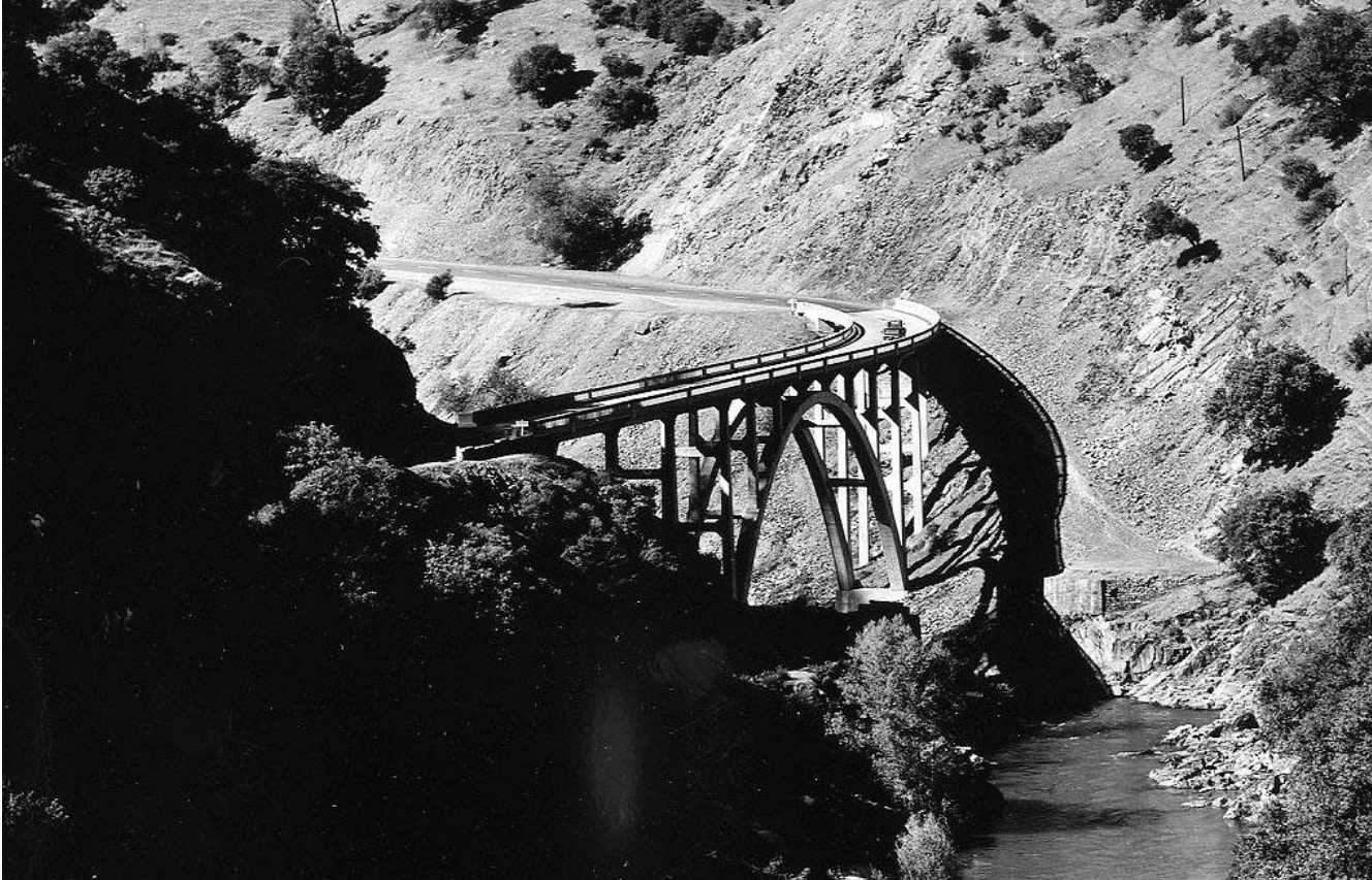
1930 West Branch Bridge
