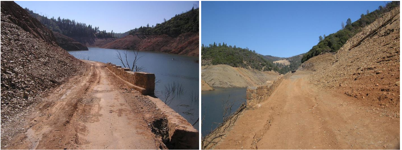
Beautiful stone masonry under water during normal rainfall years
