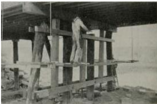
worker seen cutting bents
