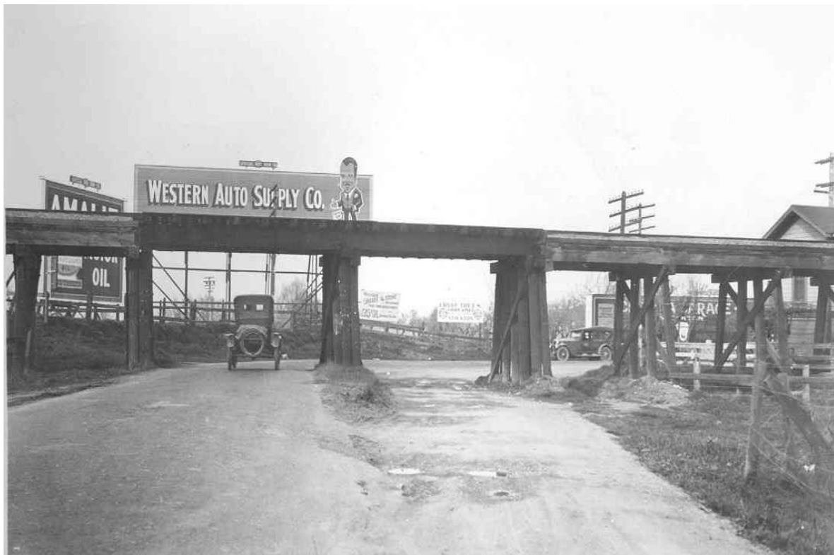
Lincoln Highway passing under trestle, 1925. Right opening was for trucks and wagons. Caltrans photo
