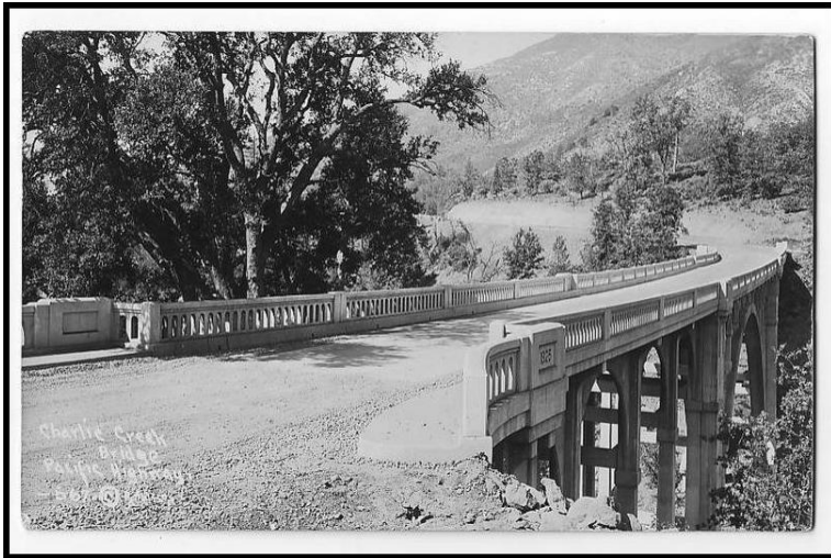
1925 Charlie Creek Bridge
