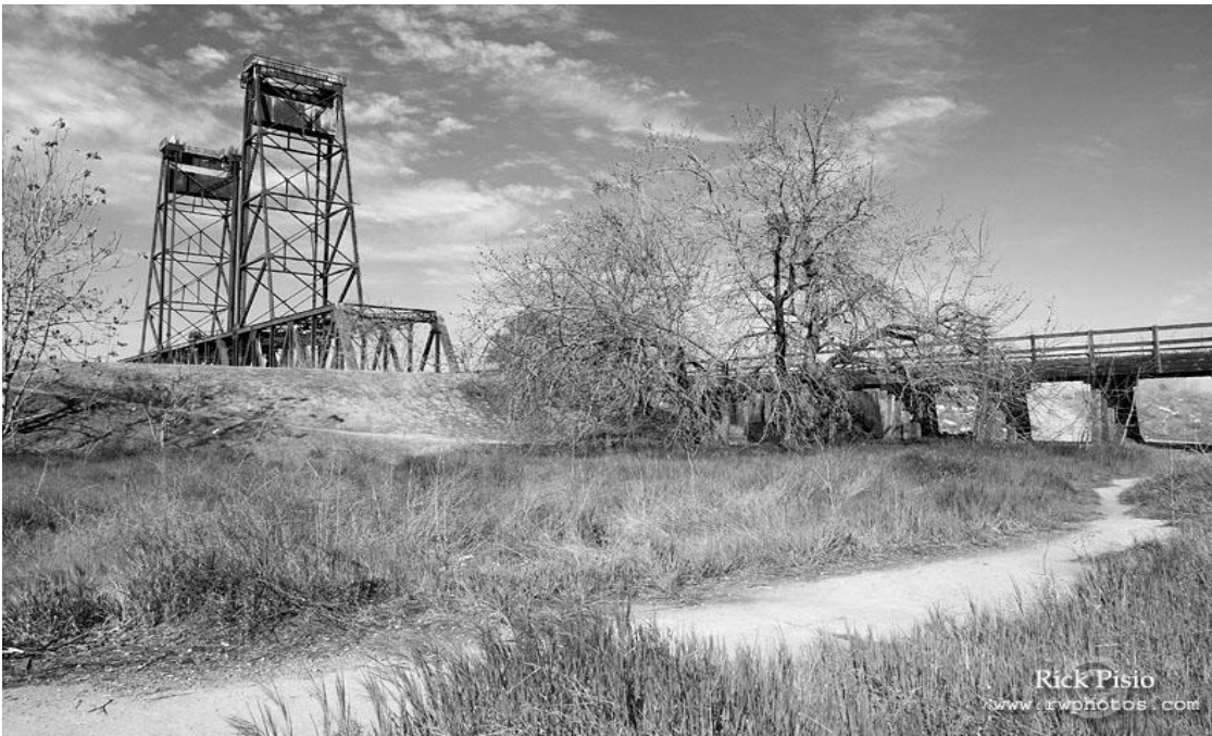
The 1895 iron truss bridge ?
