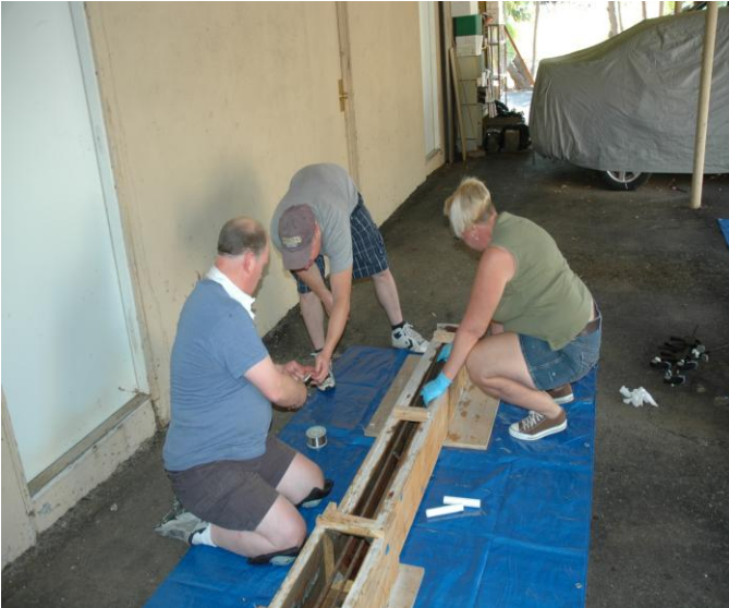
Joel, Gregg and Jackie installing rebar and preparing to fill with cement
