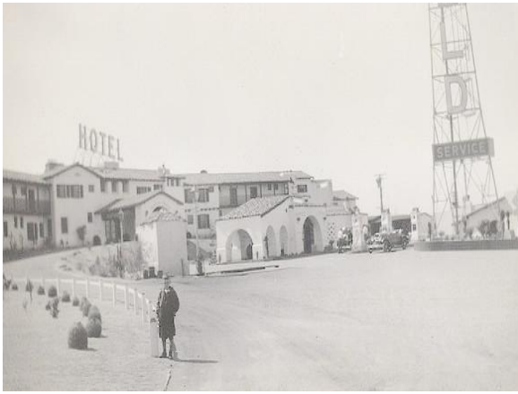
Example of California station (Route 66 Barstow)
