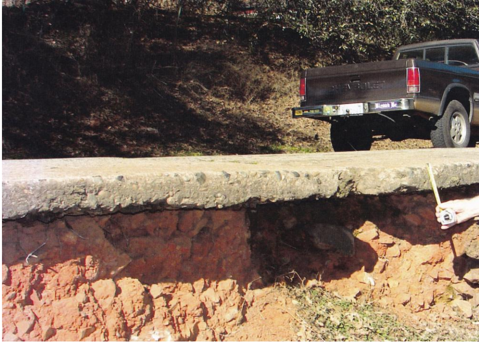
Original 1917 Lincoln Highway Concrete
