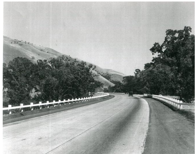
SB Grapevine Canyon JNO Grapevine Creek Bridge
