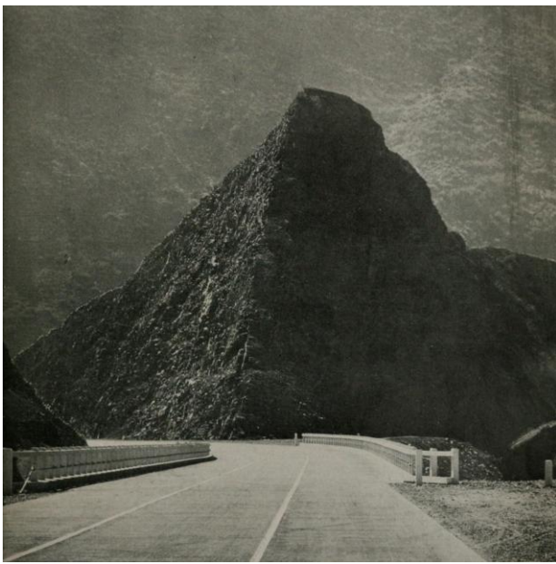
SB 1933 Piru Creek Bridge & Pyramid Rock
