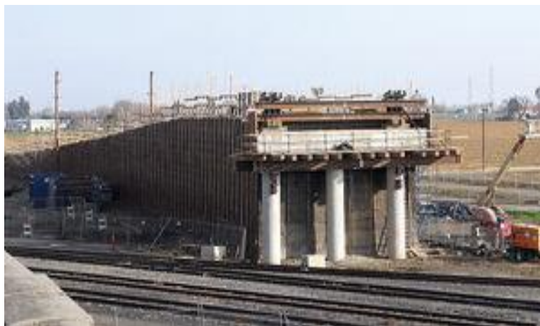
Work in progress on by-pass
