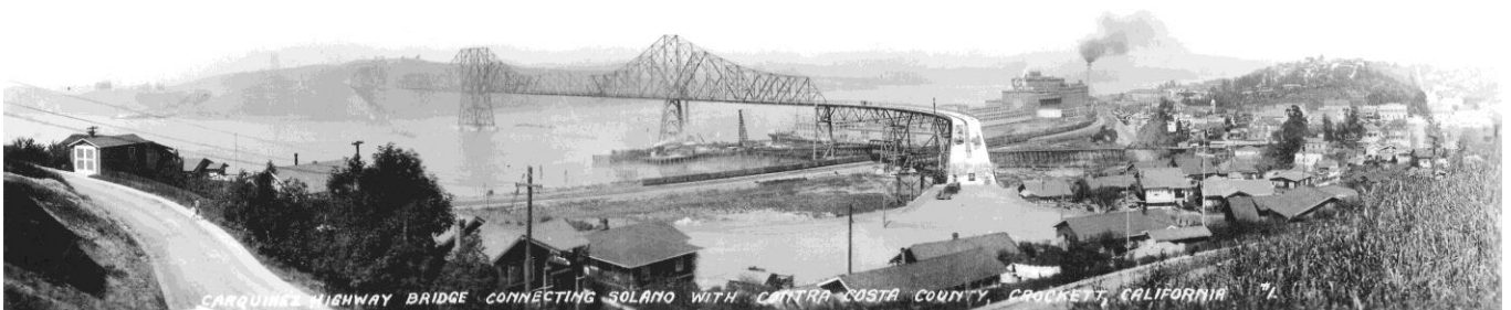
Traffic moving across recently opened bridge
