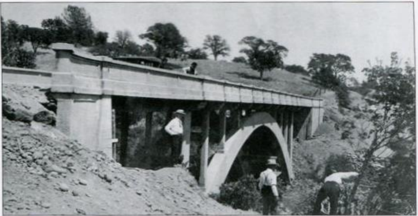
Pictured here in 1915, the Orangevale Avenue Bridge, a reinforced-concrete structure designed to last approximately 50 years, has serviced the community for more than 90 years and allows Orangevale residents and visitors to traverse Orangevale's beautiful rolling hills. (Courtesy SAMCC, No. 77/35/500 and No. 77/35/481.)
