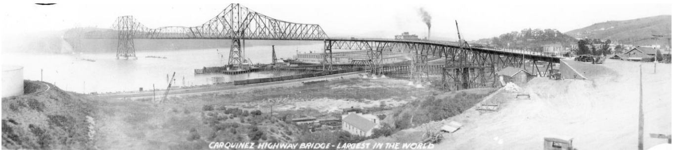
Bridge near completion 1927
