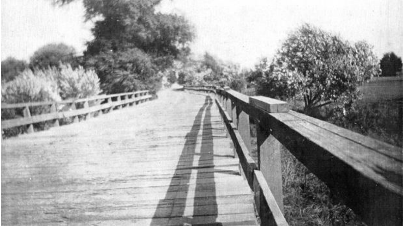
Dry Creek Bridge on Lower Sacramento Road South of Galt
