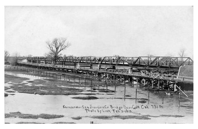
Photo dated February 5, 1910 showing temporary bridge used during construction of steel truss bridge seen in background.
