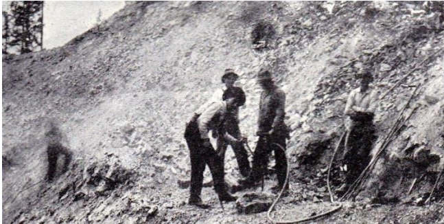
Drilling and Blasting
