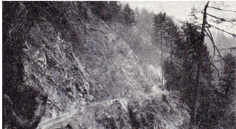
Completed road around precipitous mountain side
