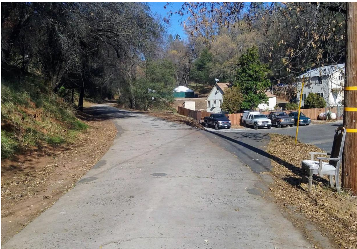
Longest stretch of Lincoln Highway concrete in Placerville, approx. \frac{1}{4} mile in length. Looking up-hill approx. 500 yds. below preceding photo. It climbs up-hill and turns to the right and continues to climb until reaching above photo. Horseshoe curve followed contour of old canyon which would be later filled for new alignment of Placerville Dr.
