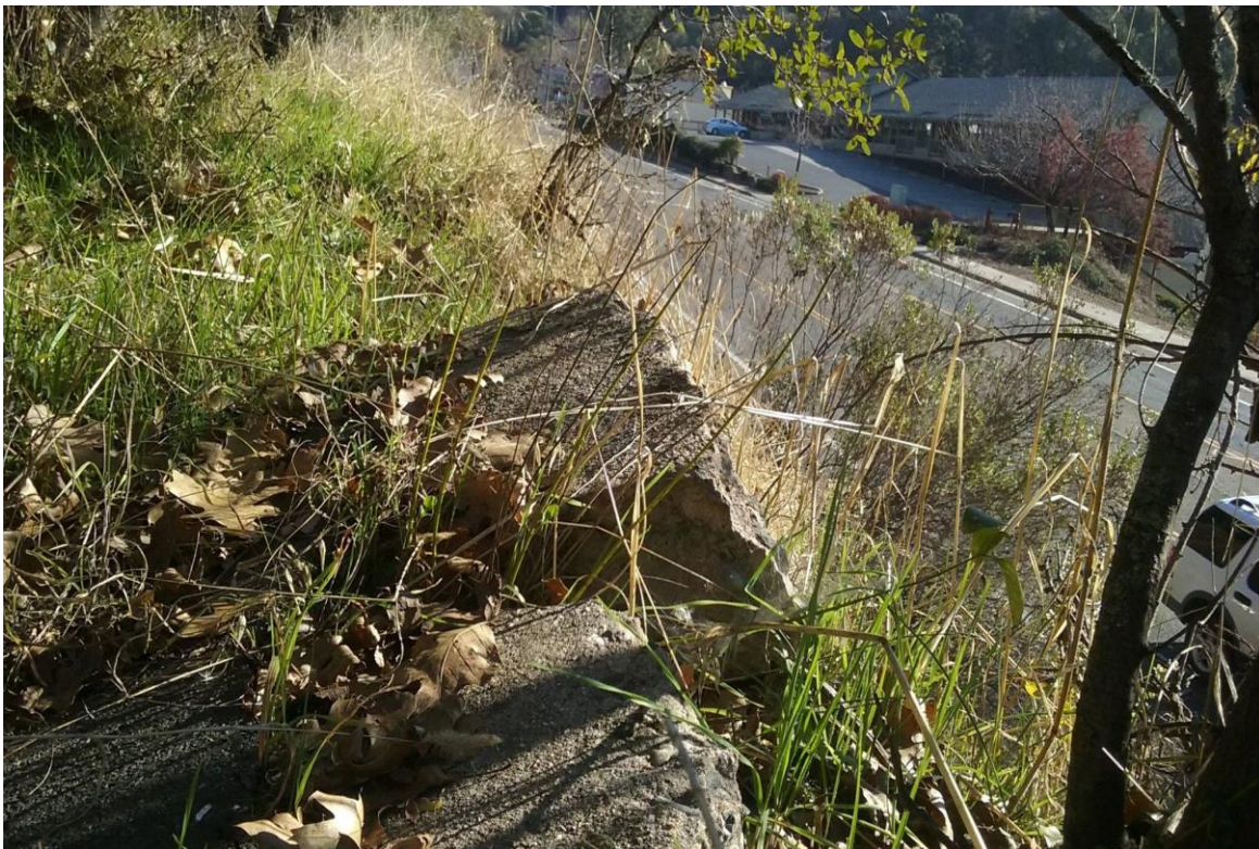
Remnants of old highway located above Placerville Dr. appear to be approx. 6 in thick
