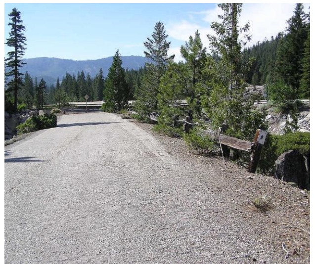
Old wooden and cable barrier railing
