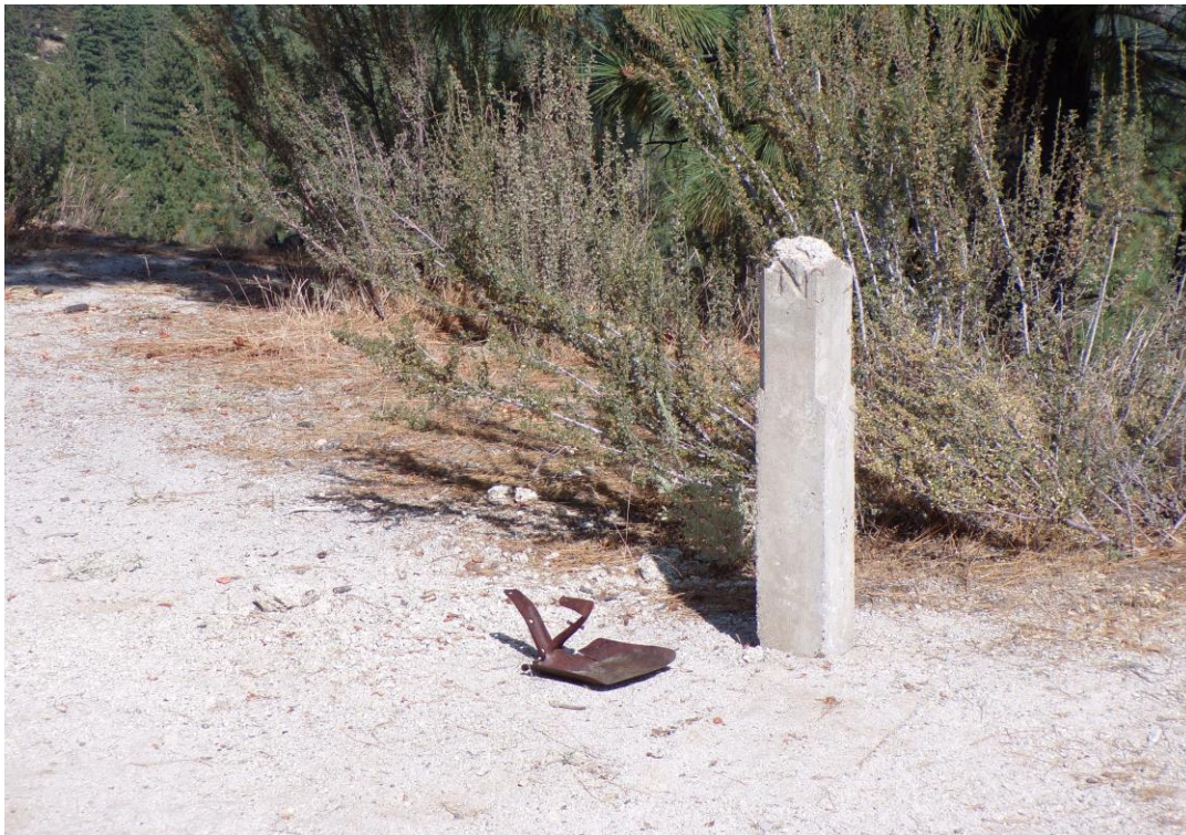
Nevada Highway Marker with broken head. Shovel head was found several feet off the road
