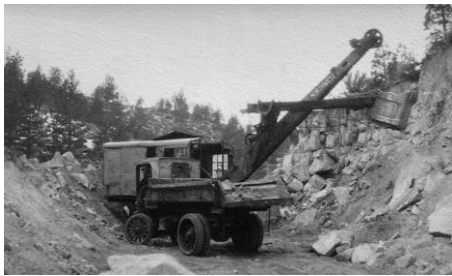
Steam Shovel digging out a highway cut 1926
