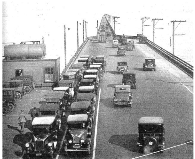
Staging area at foot of Pier 1927
